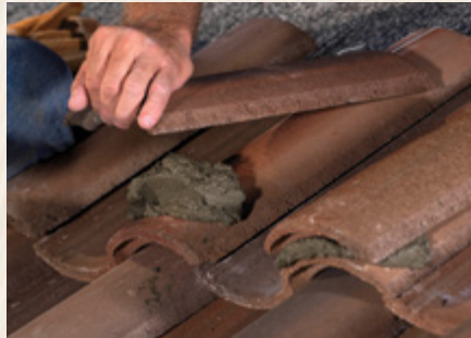
Placing The Mortar
