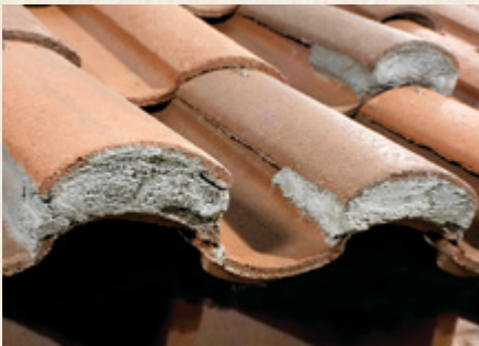
Close-Up of Boosted Eave
