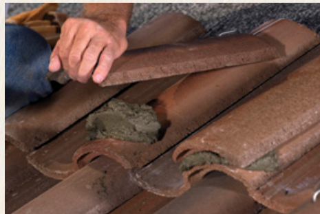
Placing The Mortar
