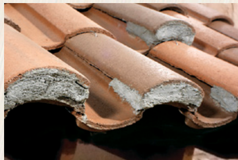
Close-Up of Boosted Eave
